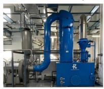
The slurry is then separated, and the liquid can be recycled or treated, while the captured particulate matter is disposed of or further processed if necessary.
